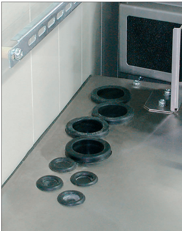
Cable entry made of rubber gland seals
