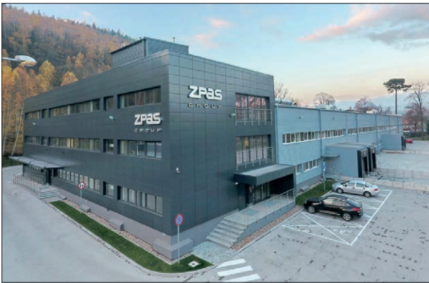
Nowa Ruda – Drogosław, Piłsudskiego Street Manufacturing plant – electrical assembly
